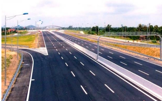
Street lights in Phu Giao District
